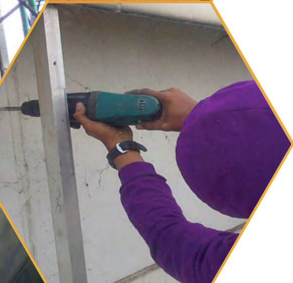
Pemasangan Aluminium Composite Panel (ACP)
