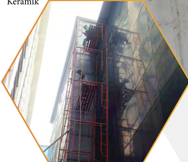
Pemasangan Aluminium Composite Panel (ACP)
