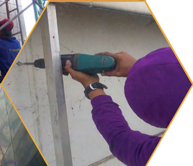
Pemasangan Aluminium Composite Panel (ACP)
